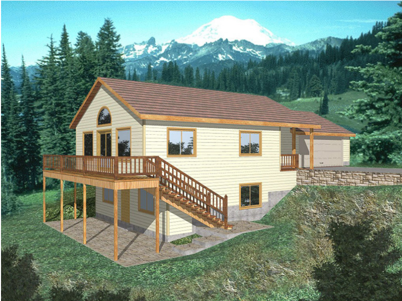
TWO LEVEL: Full story drop in site
